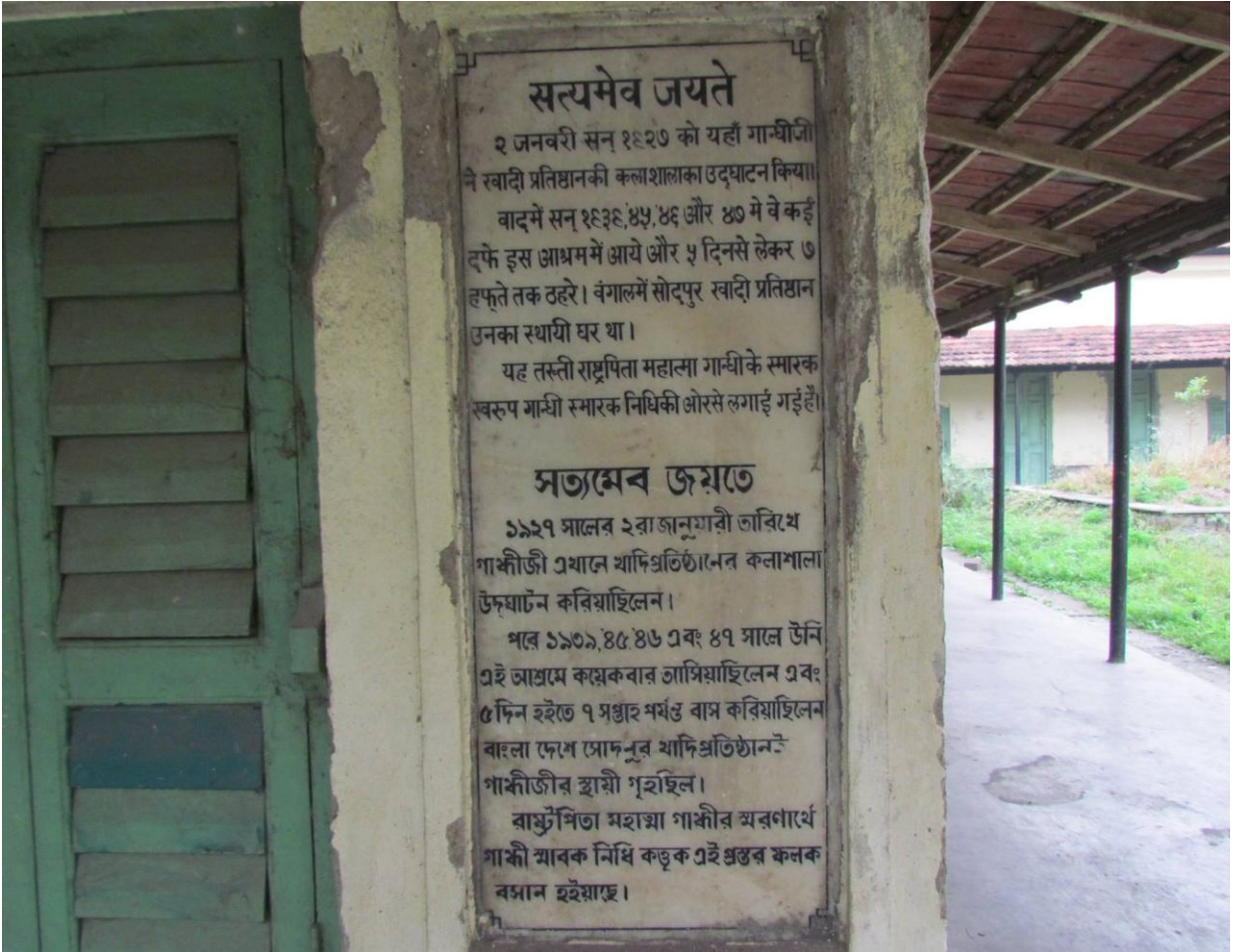
Plate 73 & 74 – Sodepur Khadi Pratisthan , present condition
